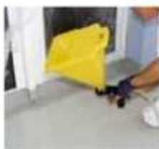
13 ... wdmuchać Triflex Micro Chips.
