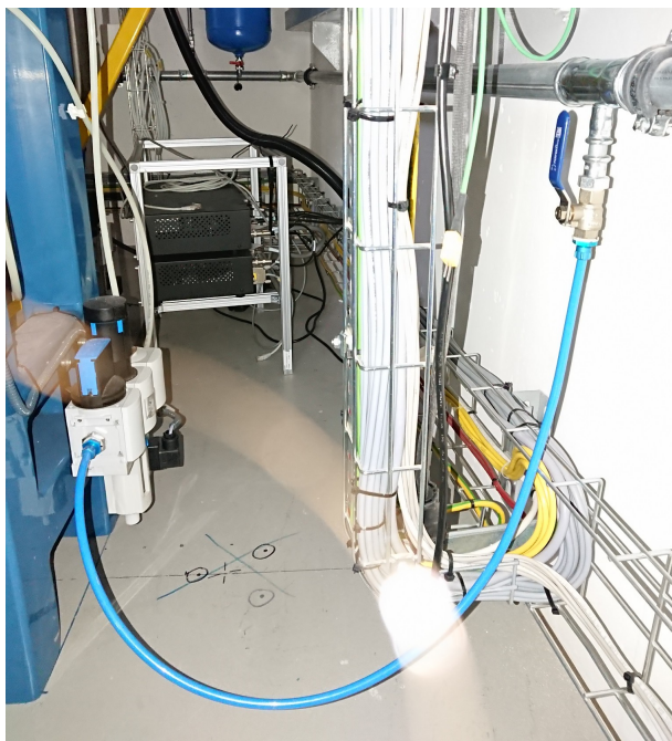
Pic. 1. Connection between a backbone connection and a supply manifold
